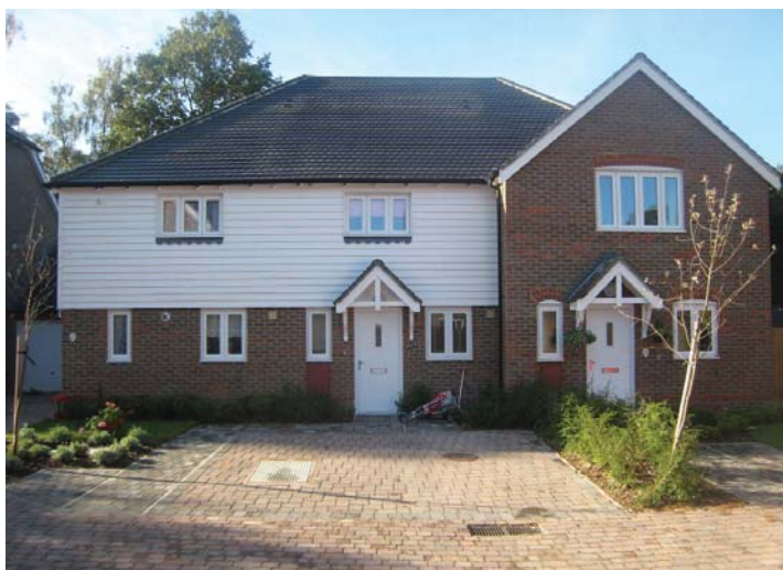
Completed Units at Gwynne Gardens
