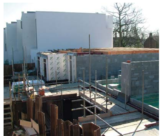
Under construction - Phase 2 of Queensmere Road
