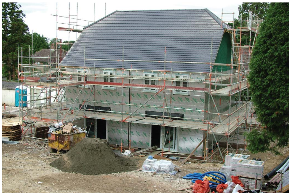
Units at Gwynne Gardens East Grinstead East Sussex for Hillreed Homes
